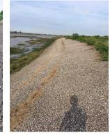
new concrete blocks would not remove this challenge, whereas OSA ensures the revetment is one single material. OSA is also quicker to lay than concrete blocks meaning that the project will be on-site for less time than if concrete blocks were proposed. There are also significant challenges installing concrete blocks in a tidal environment alongside modern health and safety standards.
